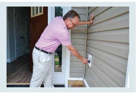
There is an outside GFCI outlet with a reset button, typically located in the garage, but may be elsewhere on the exterior of your home. It controls power to garage and outside receptacles.
