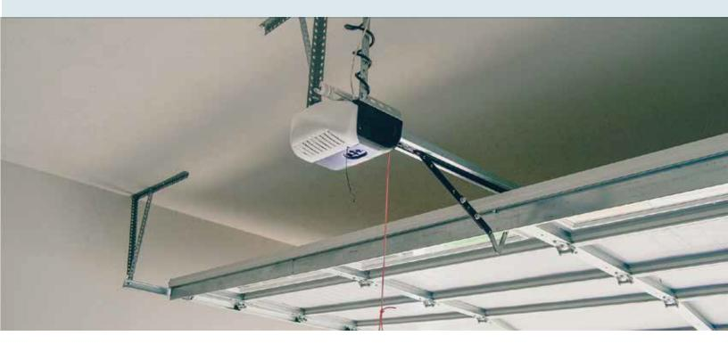
You get two garage remotes at closing with your closing package. There is wire hanging from garage door motor, this is the antenna for your remotes and needs to be in good standing for your garage remotes to work properly. Do not cut or damage this wire. Your garage remotes are battery powered; you may need to change these batteries from time to time. If you need to obtain a replacement garage remote, you may purchase one from our vendor or a local hardware store that has them in-stock.
