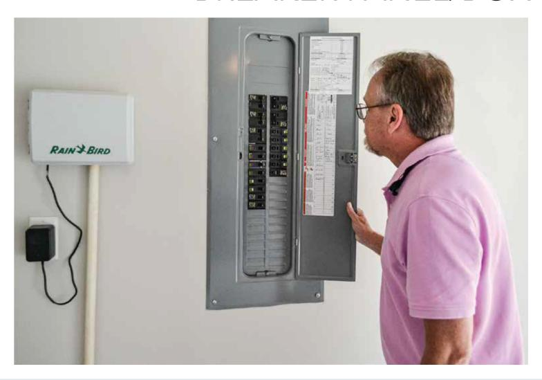
We label all break panel/box switches once electrical is installed. If one breaker trips turn it off and then back on. You can tell the breaker is tripped when it is not in an "on" or "off" position, but rather in between.
